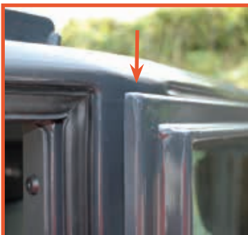
Accurate grinding of welded parts and cab bars.
